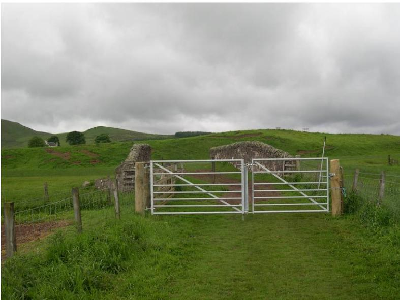
*A Centrewire 2-in-1 gate at the march boundary alleviates any worry about stock straying onto the road or adjacent golf course, whilst still allowing multi-use access. The other half of the gate is usually locked to restrict illegal vehicular access, but the gate can be opened full width when required for farm access.*
